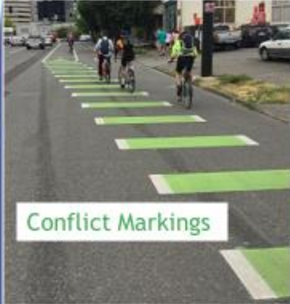
Visually narrow road (slows traffic)
