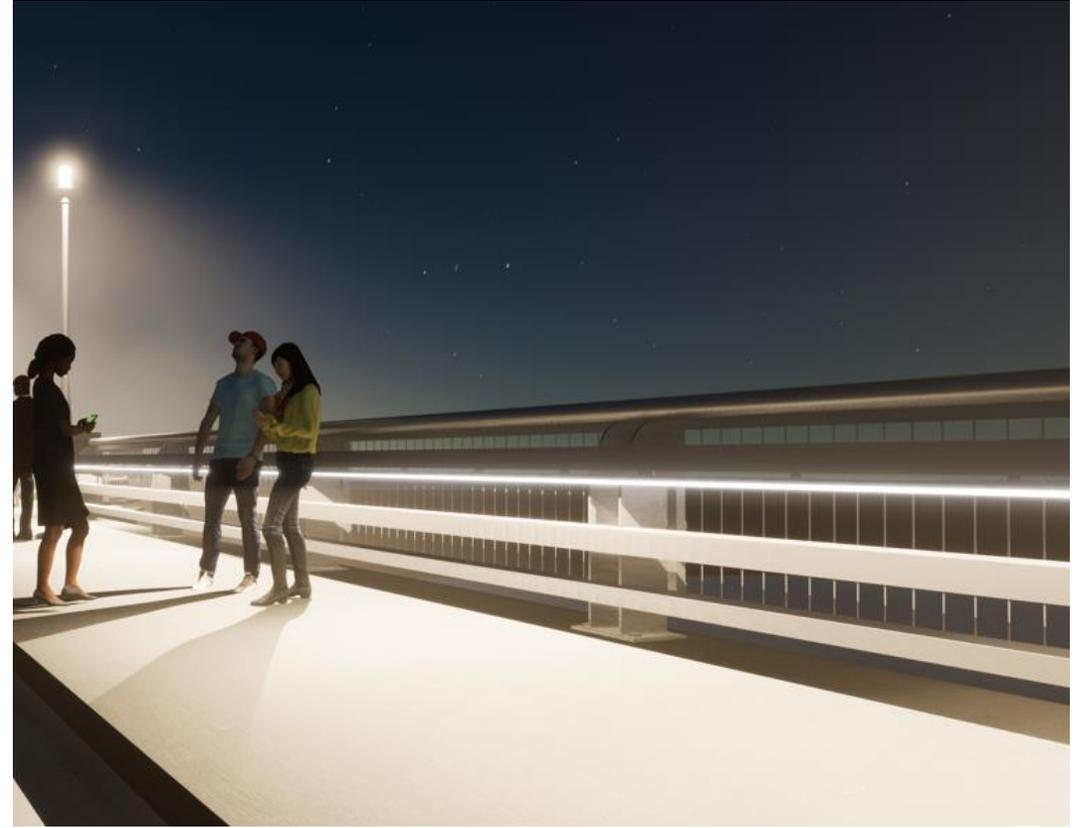
Bridge Rail Option 2 Metal Vehicular Bridge Rail/Metal Pedestrian Fence, Under Top Rail Lighting
