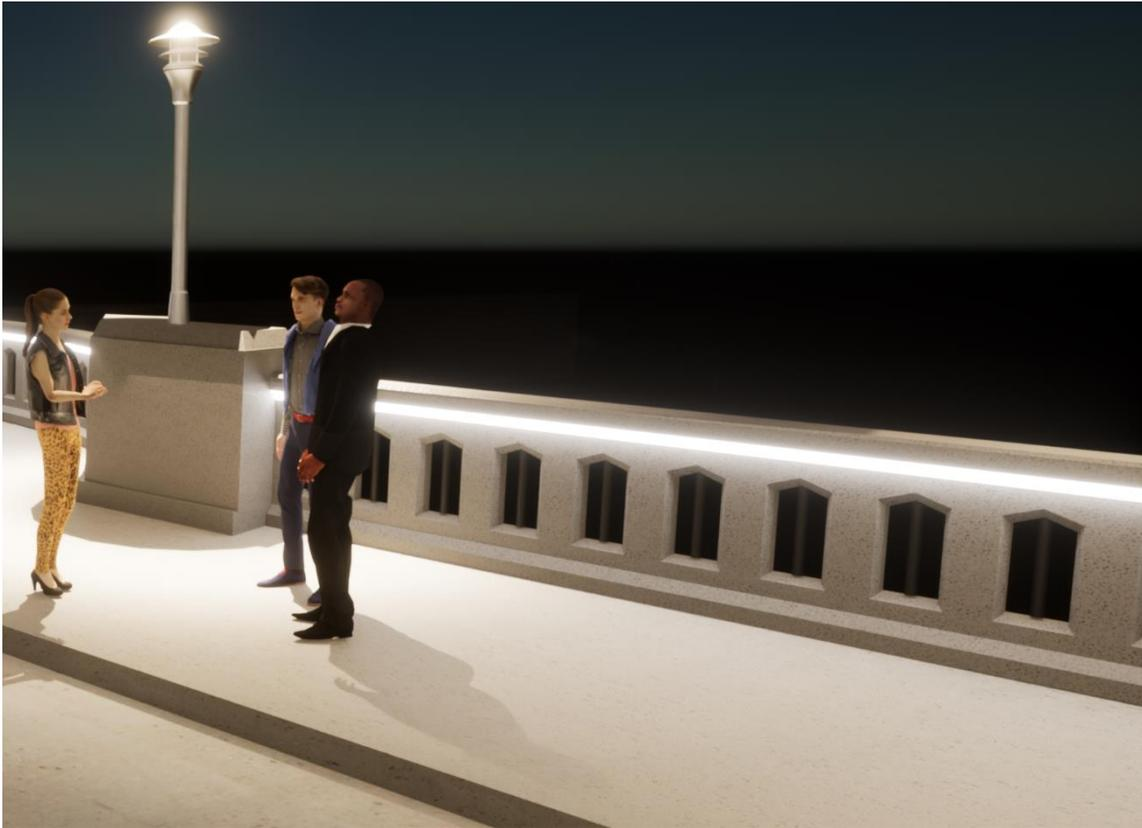
Bridge Rail Option 1 Concrete Vehicular Bridge Rail, with Under Top Rail Lighting
