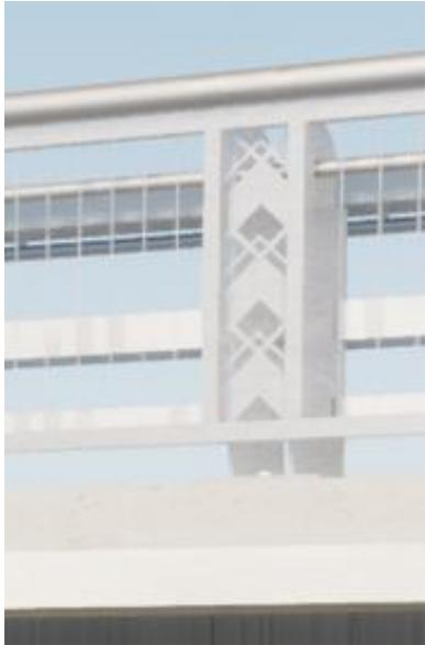
Option 2A - Metal Vehicular Bridge Rail with Metal Pedestrian Fence at Overlook - Layered
