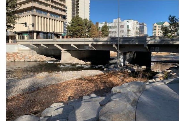
VIEW OF NORTHERN BRIDGE
