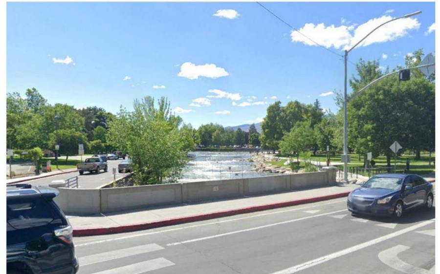
SOUTHERN BRIDGE SECTION, LOOKING WEST
