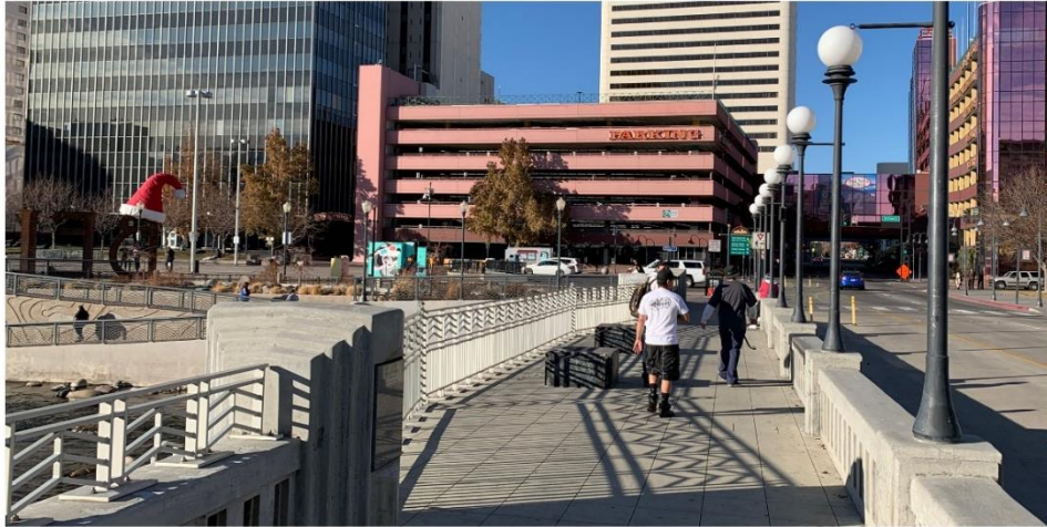
CENTER STREET BRIDGE DOUBLE RAILING - AVOID
