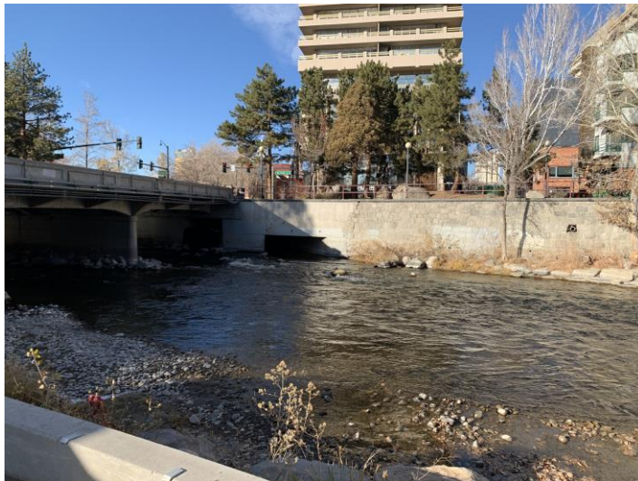
EXISTING FLOOD WALL
