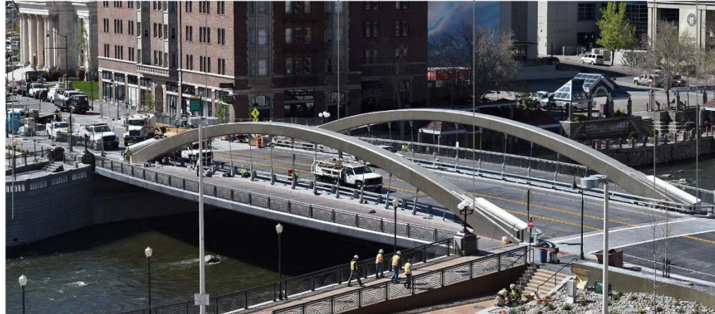
VIEW OF BRIDGE
