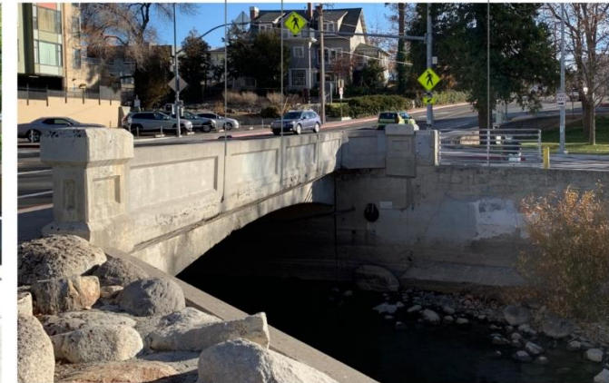
VIEW OF SOUTHERN BRIDGE
