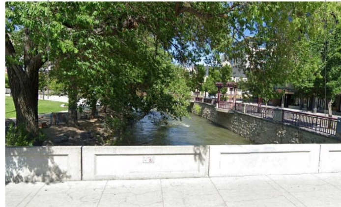
SOUTHERN BRIDGE SECTION, LOOKING EAST
