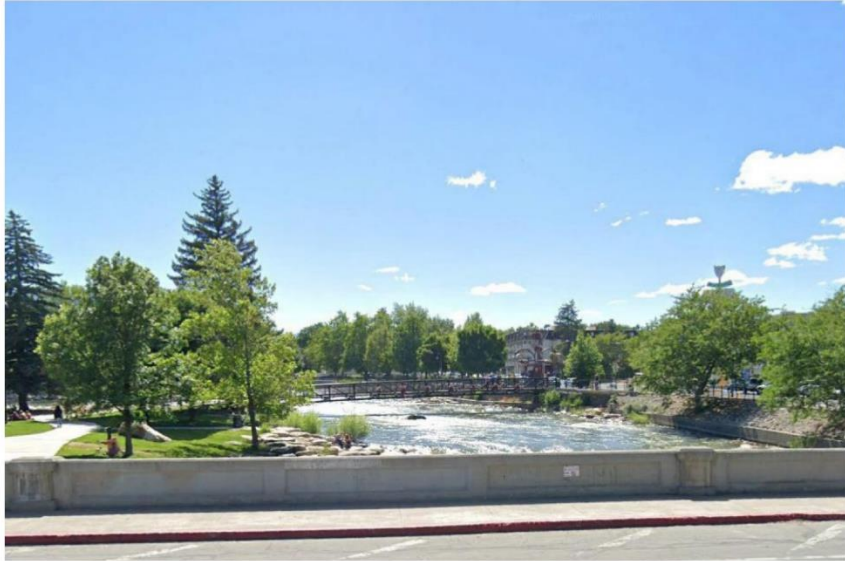
NORTHERN BRIDGE SECTION, LOOKING WEST
