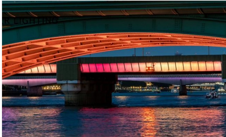
UNDER BRIDGE LIGHTING
