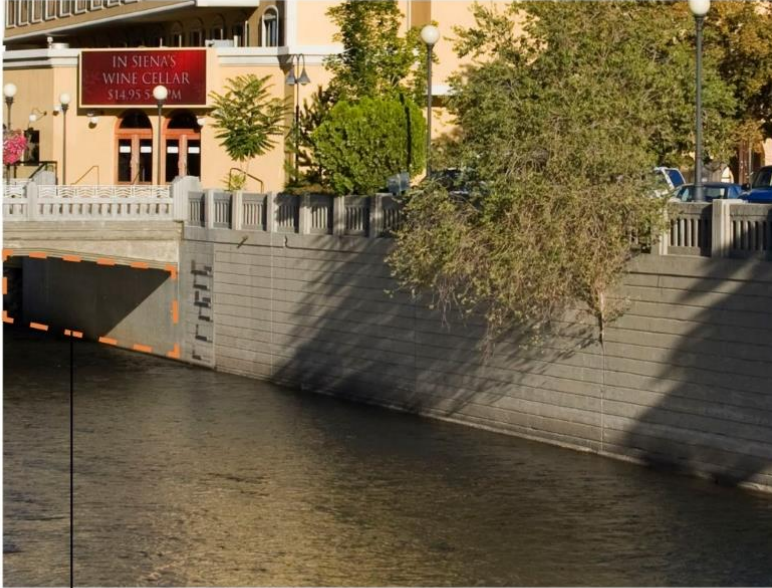
FORMLINER PATTERN FOR ABUTMENT WALL
