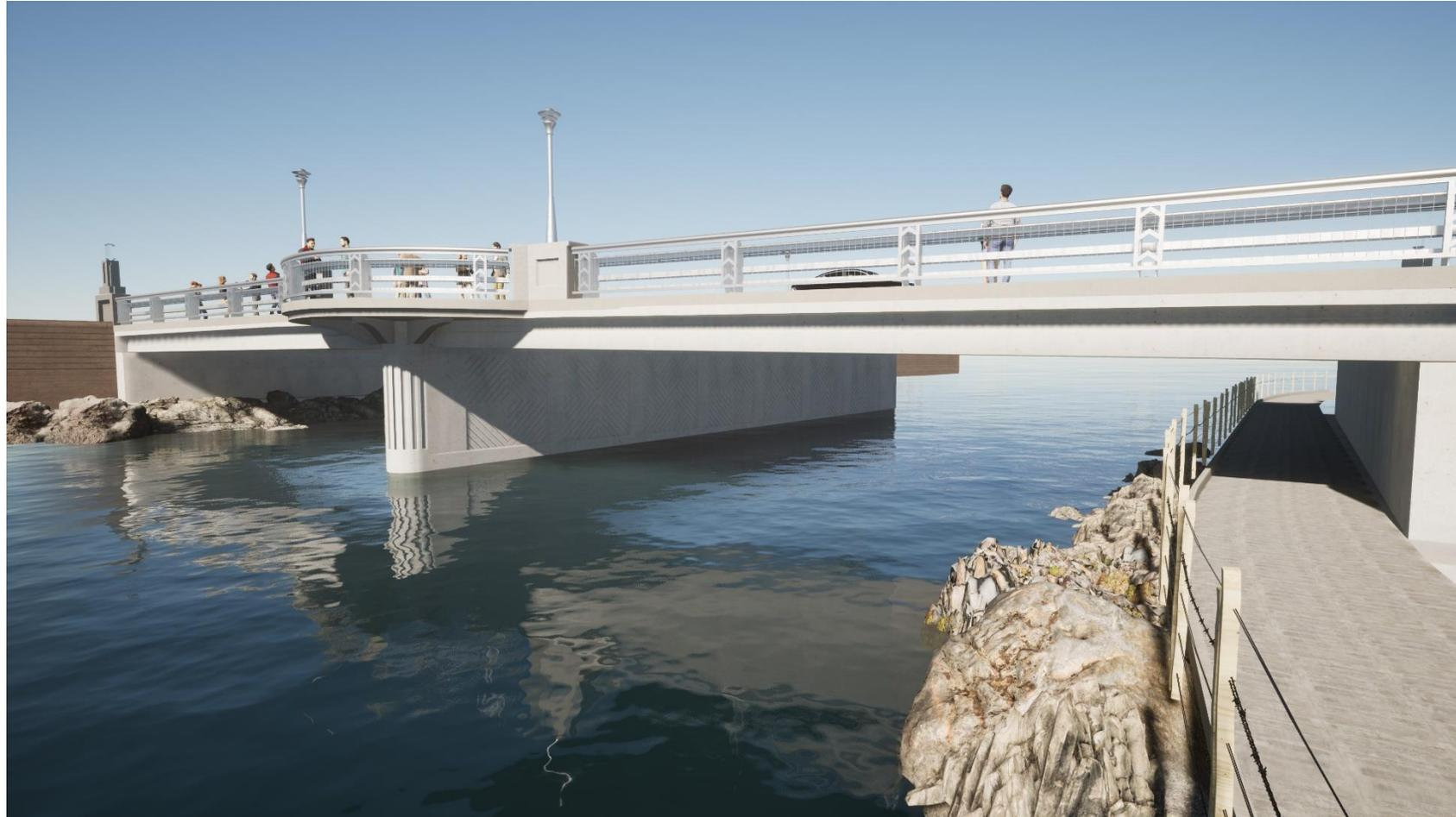
Overall Bridge Option 2 - Metal Vehicular Bridge Rail with Metal Pedestrian Fence
