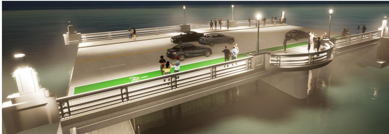
End Pylon Option 2 with Custom Luminaires and Forms+Surfaces LED Post-Top Luminaire on Mid-Bridge Pilasters and Under Top Rail Lighting
