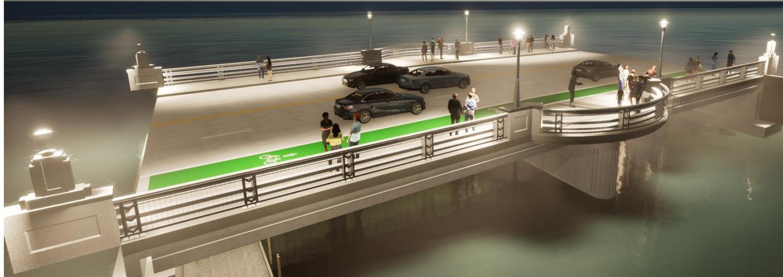
End Pylon Option 3 with Custom Luminaires and Forms+Surfaces LED Post-Top Luminaire on Mid-Bridge Pilasters and Under Top Rail Lighting
