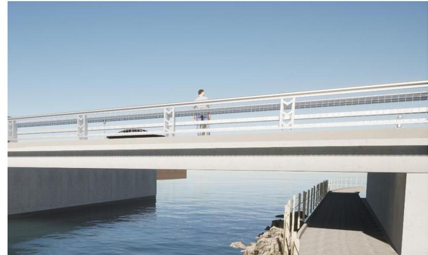
Option 2B - Metal Vehicular Bridge Rail with Metal Pedestrian Fence - Chevrons Down
