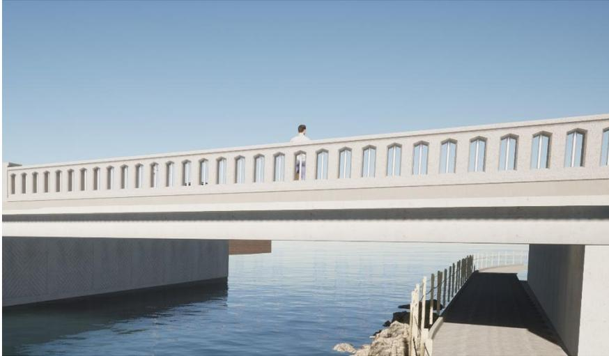
Option 1 - Texas DOT Concrete Bridge Rail/Parapet
