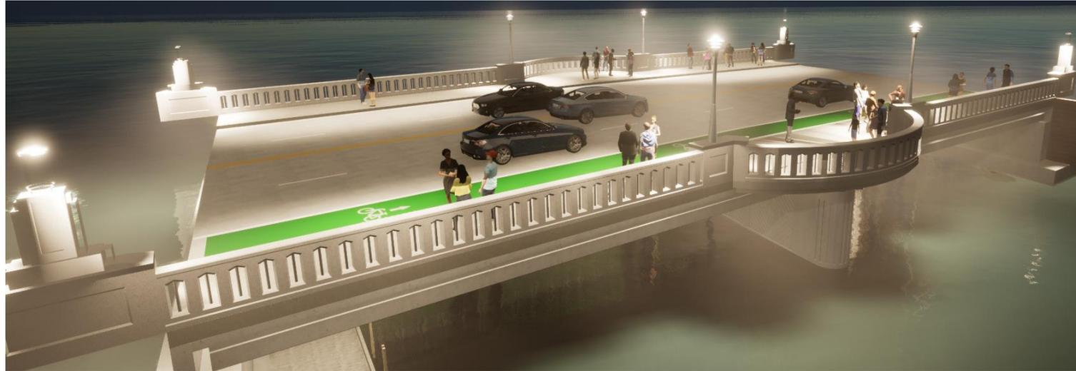
End Pylon Option 1 with Custom Luminaires and Forms+Surfaces LED Post-Top Luminaire on Mid-Bridge Pilasters
